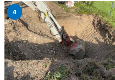
4 Digging the hole
